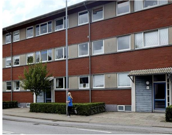
Facade of the 3-floor building.
